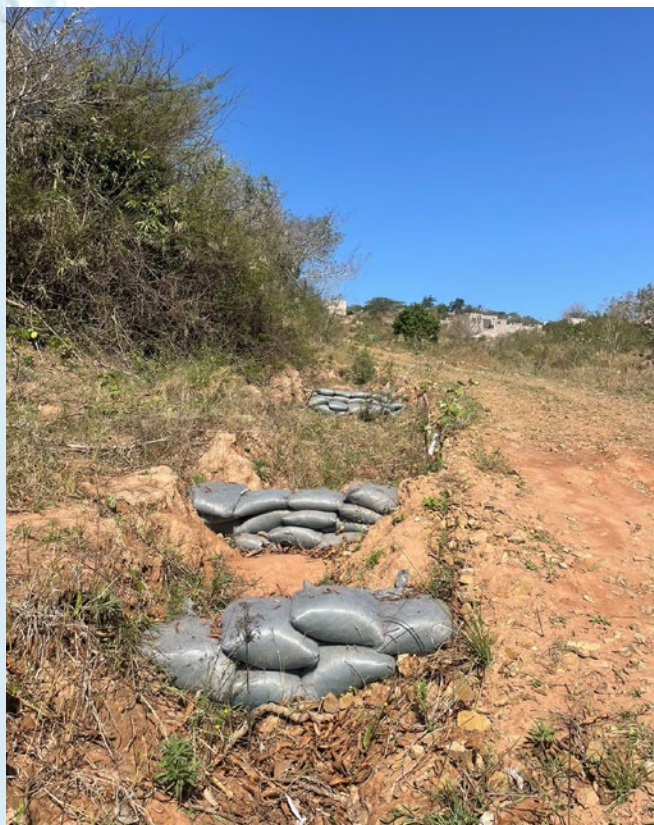
The use of sandbags as one of the erosion control measures in our Hazelmere sites.
