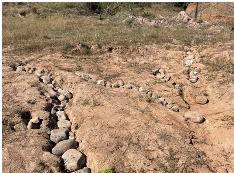
Stone-packing as an erosion control method to slow and divert water flow.
